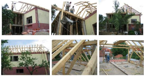
As you can see on the photos the main focus during the last week was to complete the roof. What we have done is that the we raised the timbers a bit higher than normal and we got a large space on the attic. It can be used as a place where children can sleep during summer camps.
